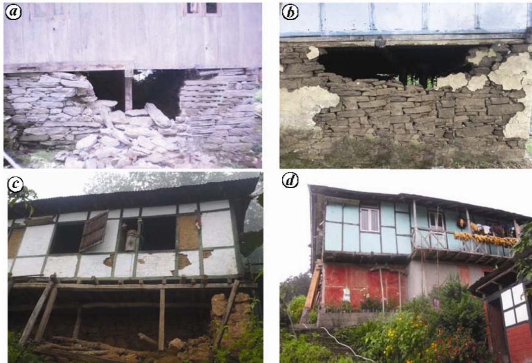
Figure 4. Partially collapsed load-bearing stone masonry wall supporting light-weight bamboo/wooden house with CGI sheet roof. a, b , House with ( a ) wooden walls and ( b ) with bamboo and wooden frame. c, d , Retrofitting with wooden posts.
